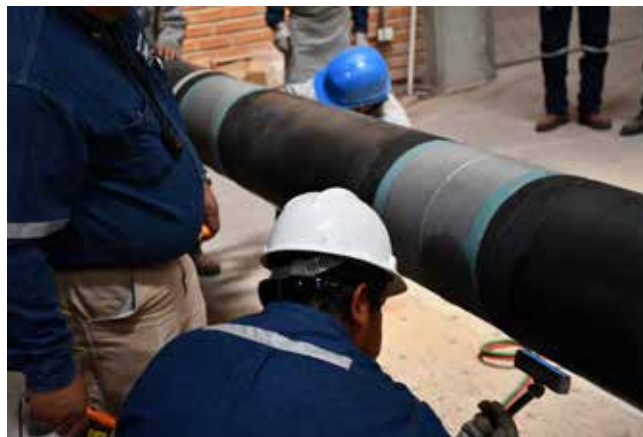
Figure 4. Treatment of PE coating using Flynn Burner head.
